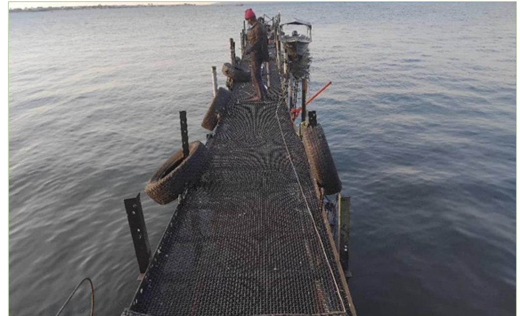
Pier before reinforcement with extra galvanized poles in the edges and adding an additional layer.
