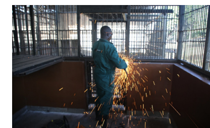
Reinforcement of the bars in the medical ward
