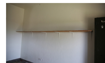
Treatment room of the medical ward
