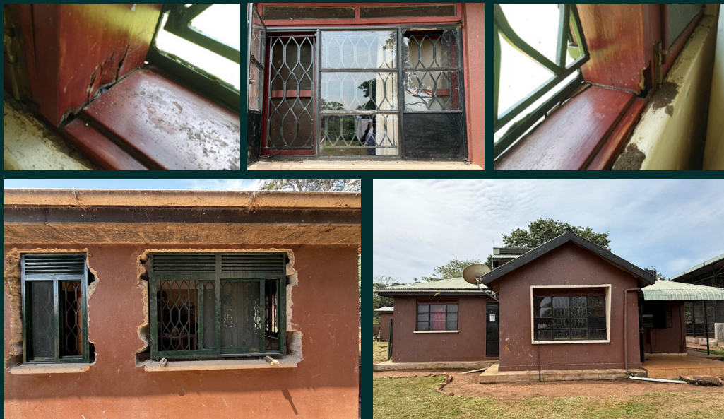
Work done on the resource centre
