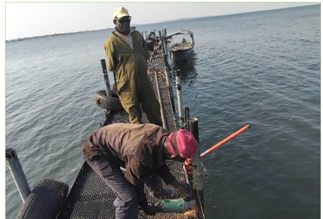
Works done on the pier; re-enforcing the edges of the pier
