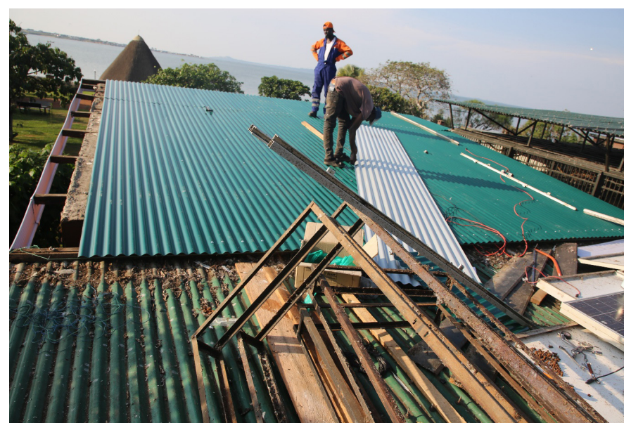
Reroofing of the medical ward
